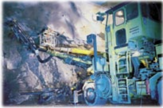
■ Pre-injection with Rheocem® 800 at Arlandabanen
