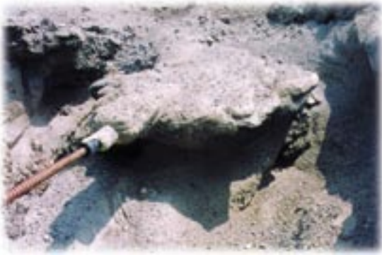
■ Sand stabilisation with Acrylic resin
