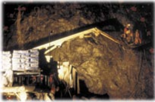
■ Rock injection with Rheocem®
